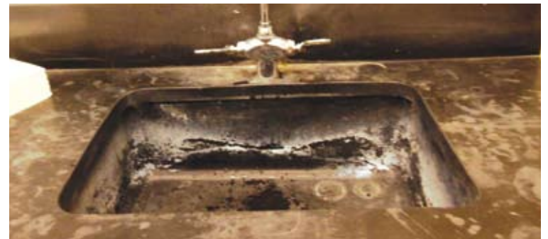
CHS sink in the Chemistry lab, the class produces college ready technicians, yet students do not have the opportunity to practice.
