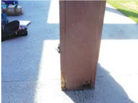
Termite damage at Whitney High.
