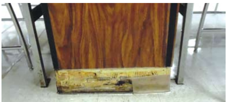
WHS desks are deteriorating and breaking apart, aisle in classrooms are so thin students must turn sideways to walk down the aisle.
