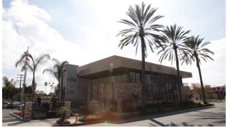
The Hawaiian Gardens Public Safety Center held its grand re-opening this past Wednesday, August 16. Photo courtesy Hawaiian Gardens.
