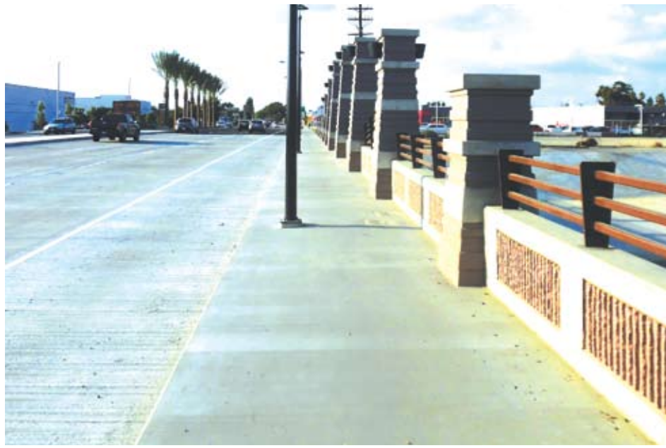
The newly finished bridge in Downey. Construction began in early 2014 and the bridge was completed in approximately 20 months at a cost of $7.3 million.
