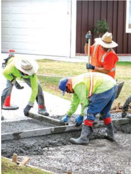
Damaged curbs, gutters, and sidewalks were removed and replaced as part of Measure I Phase 1. Construction crews pour concrete for a new sidewalk and driveway apron as part of the Measure I Phase 2 project. This area includes neighborhoods bounded by Alondra Blvd., Stage Road, Biola Ave., Rosecrans Ave., La Mirada Blvd., Ocaso Ave., Barnwall St., and Dalmatian Ave.
