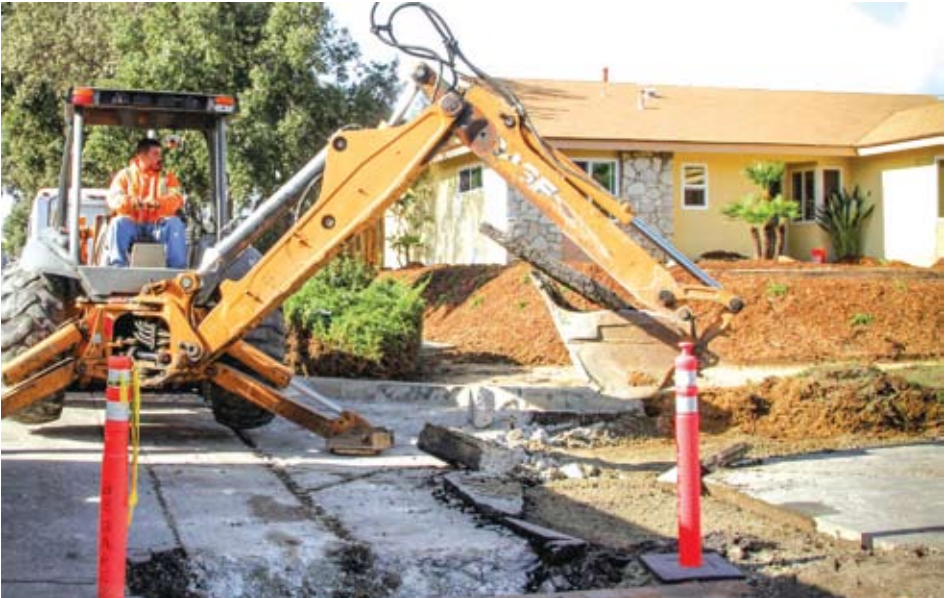
Damaged curbs, gutters, and sidewalks were removed and replaced as part of Measure I Phase 1. Construction crews pour concrete for a new sidewalk and driveway apron as part of the Measure I Phase 2 project. This area includes neighborhoods bounded by Alondra Blvd., Stage Road, Biola Ave., Rosecrans Ave., La Mirada Blvd., Ocaso Ave., Barnwall St., and Dalmatian Ave.
