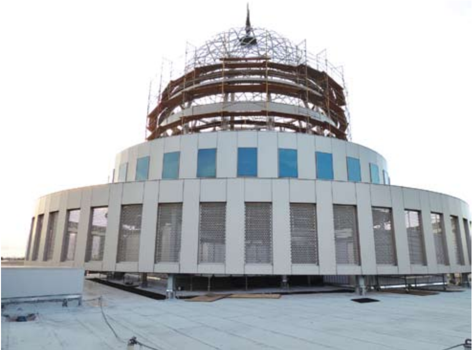
The dome on the top of the Atkinson, Andelson, Loya, Ruud & Romo building is being repainted. Representatives told HMG-CN that this happens every five years to metal structures. Photo by Eric Lee.
