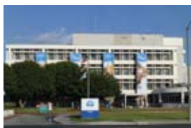
PIH Health Hospital – Downey
