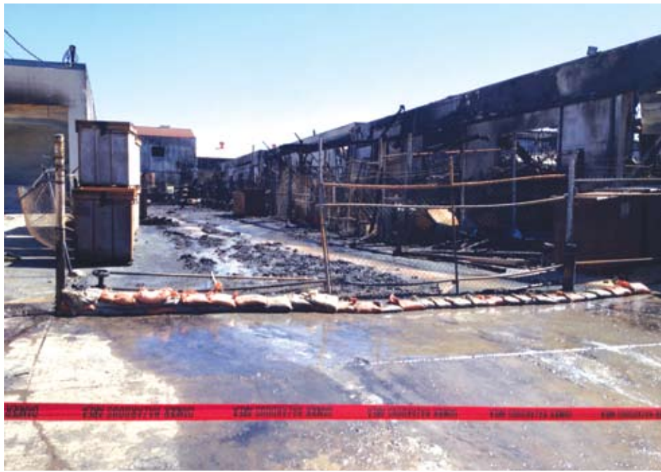
A massive set of explosions rocked the Sunshine Industrial Park in Santa Fe Springs this past Saturday afternoon at around 4:45. One hundred fire-fighters from Downey, Santa Fe Springs, LA County, Compton, and Vernon fought the four alarm fire. The explosion and fire destroyed two businesses and damaged several others. Photo by Brian Hews
