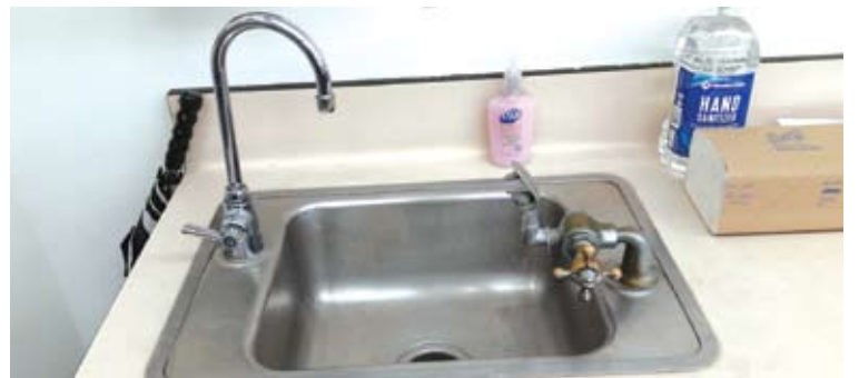
HAWAIIAN ELEMENTARY sinks and water faucets in the classrooms have not been updated since the 1970's.
