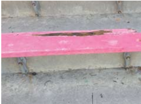
Broken bleacher seats at Artesia High.
