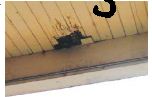
Rotting wood ceilings at Ross ES.
