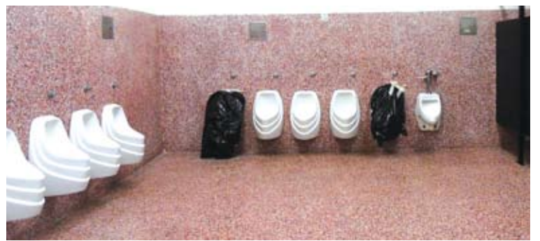
AHS has only one boys bathroom, one handicap stall and no privacy stalls; the girls bathroom stalls are in need of repair; both flood often.
