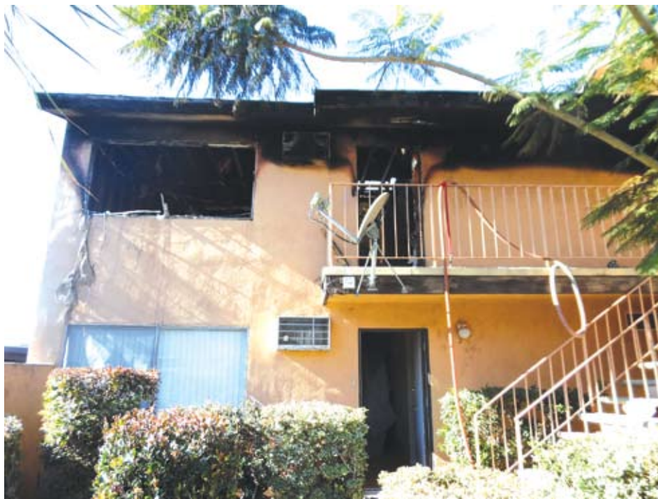
A fast moving fire ran through an apartment located at 186th and Jersey in Artesia last Saturday. 6 different stations responded to the fire, and the firefighters managed to confine the blaze to one unit. One resident was taken to hospital due to smoke inhalation. Photo by Tammye McDuff.
