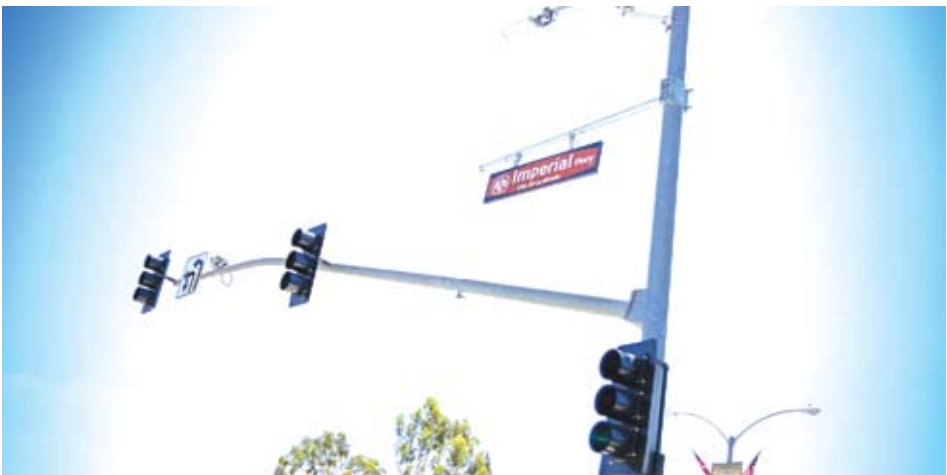
New traffic light at Imperial and Ocaso. Traffic signals were replaced due to the increasing maintenance cost of aging components.
