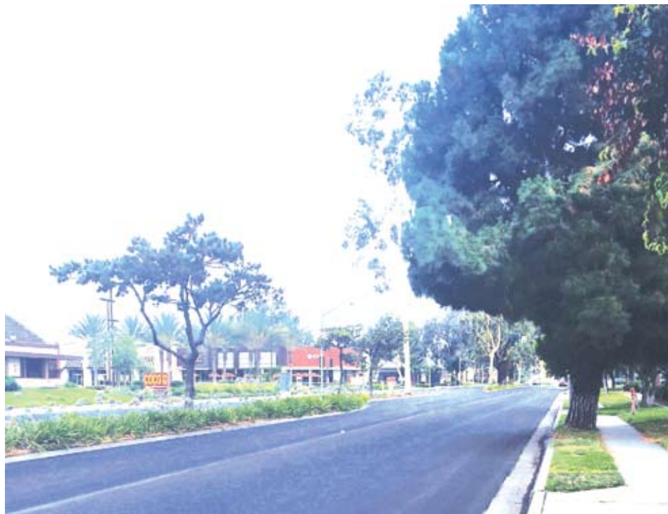
Improvements for Studebaker Road from Artesia Boulevard to Alondra Boulevard in Cerritos were completed at the end of June at a cost of $642,305. Photo courtesy city of Cerritos.
